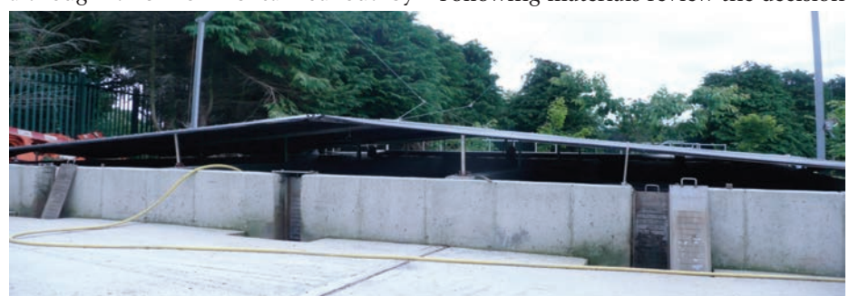
Borrisoleigh wastewater plant new dewatering beds, with decanting doors and covers
